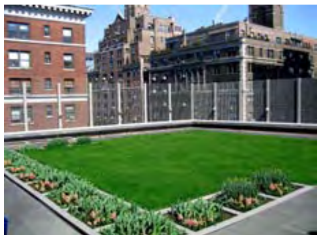
Green roofs can provide usable open space, reduce heat gain and filter urban run-off.
