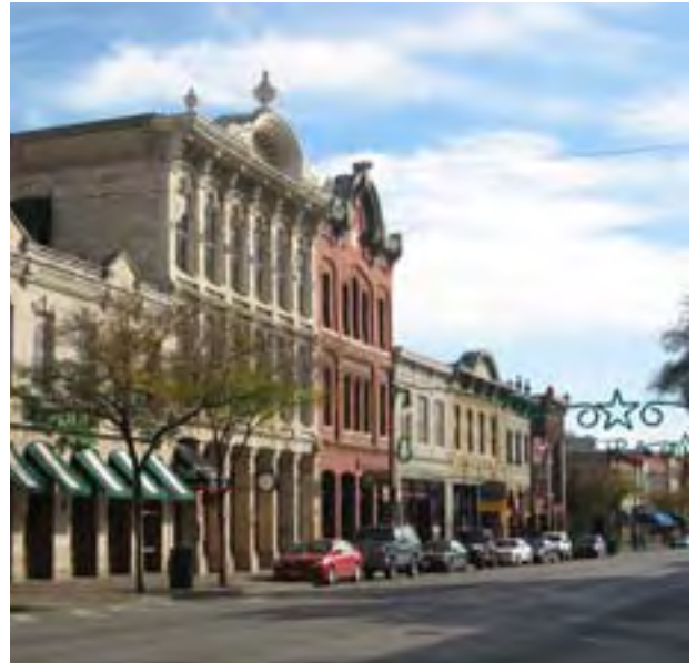
East 6th Street is Austin's most extensive district of Victorian mercantile buildings.
